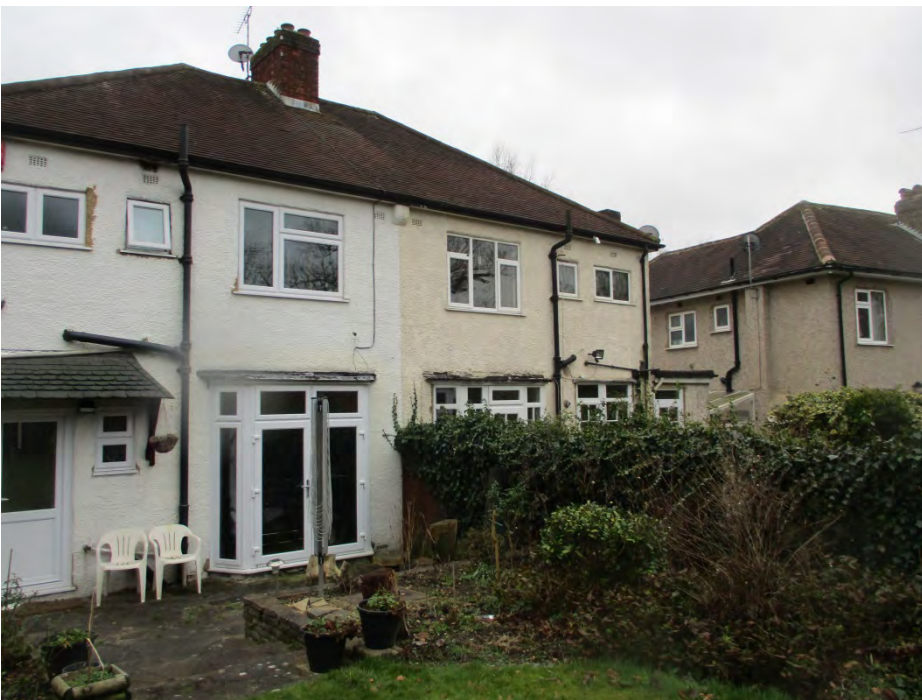
Looking towards rear of 53
